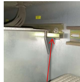
Siemens fix method of hook
